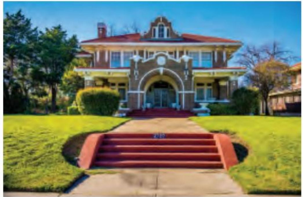
PHOTOS BY MICHAEL CAGLE, ASSOC. AIA
