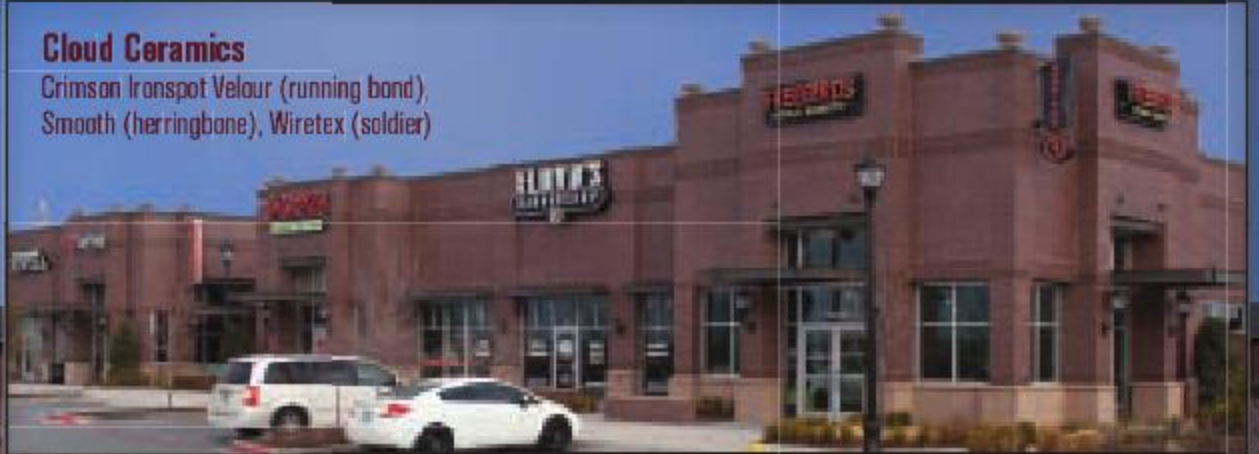
Frisco Market Center Phase I Frisco TX
