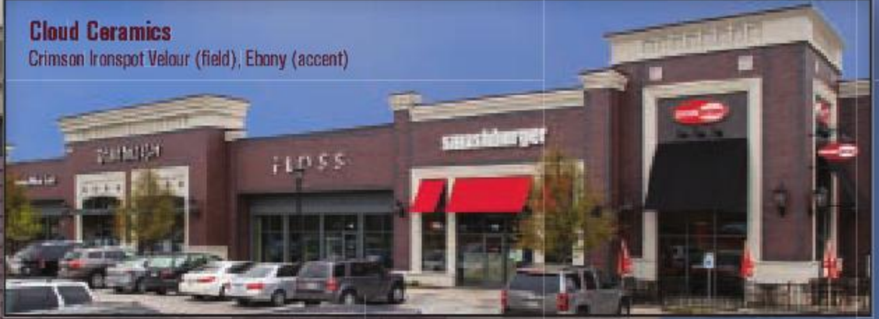
Coppel Manors Retail Center Coppel TX
