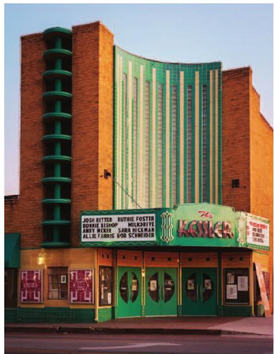
PHOTOS BY MICHAEL CAGLE, ASSOC. AIA
