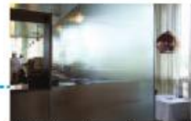
Butt-glazed storefront system with structural glass fins anchored to the floor and underside of existing wood beam. Opacifying film (Lumisty Glass Film by Sumitomo) is applied to storefront panels.
