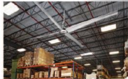
HVLS Fans Air movement to reduce energy costs and improve comfort and productivity
