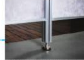
Extruded 6-inch aluminium shelf system by Rakks/Rangine with 1 2-inch L-bracket and PC-2 compression poles anchored to the floor and underside of existing wood beams.
