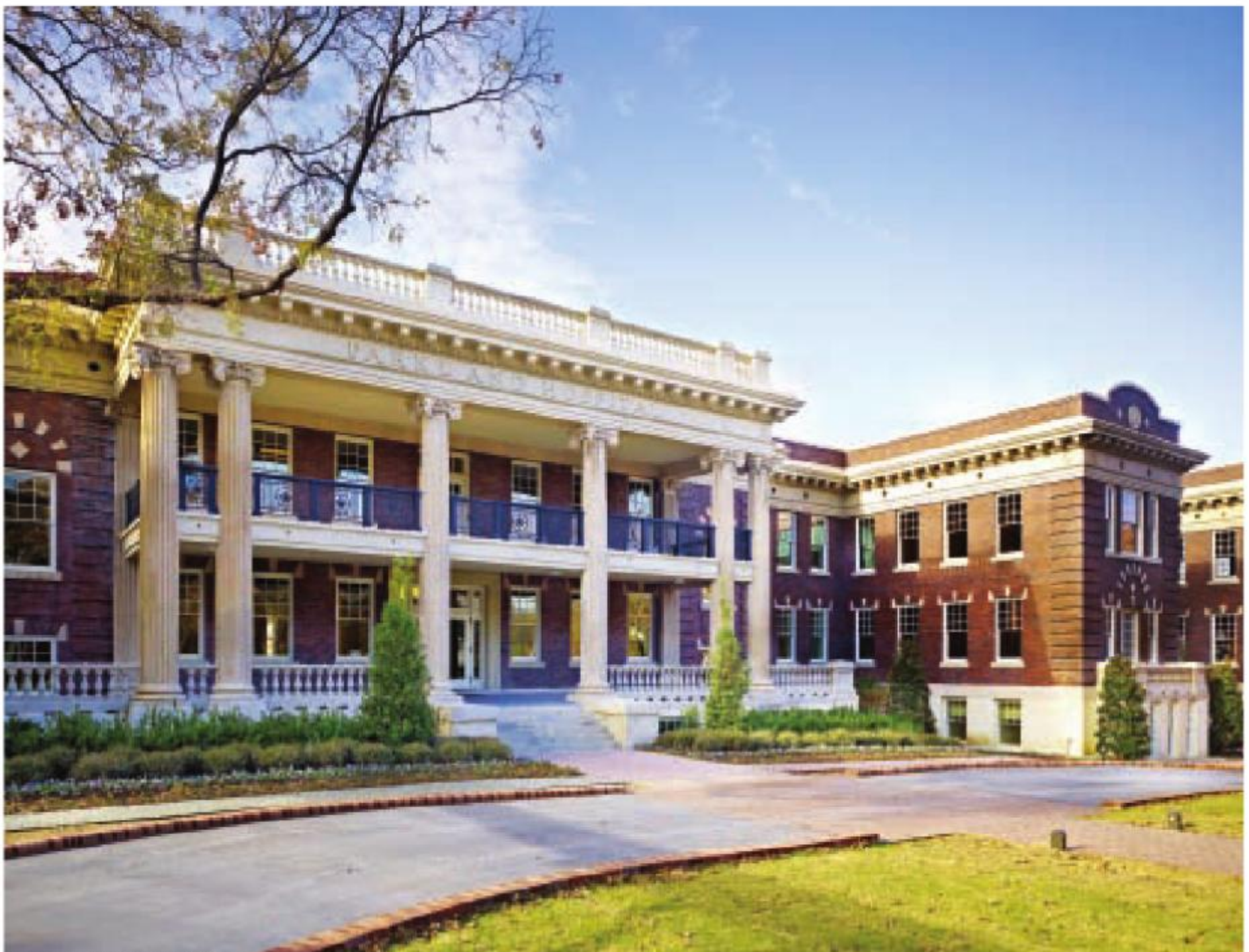
Maple Facade, 2009 - John Davis, DVDesign Group
