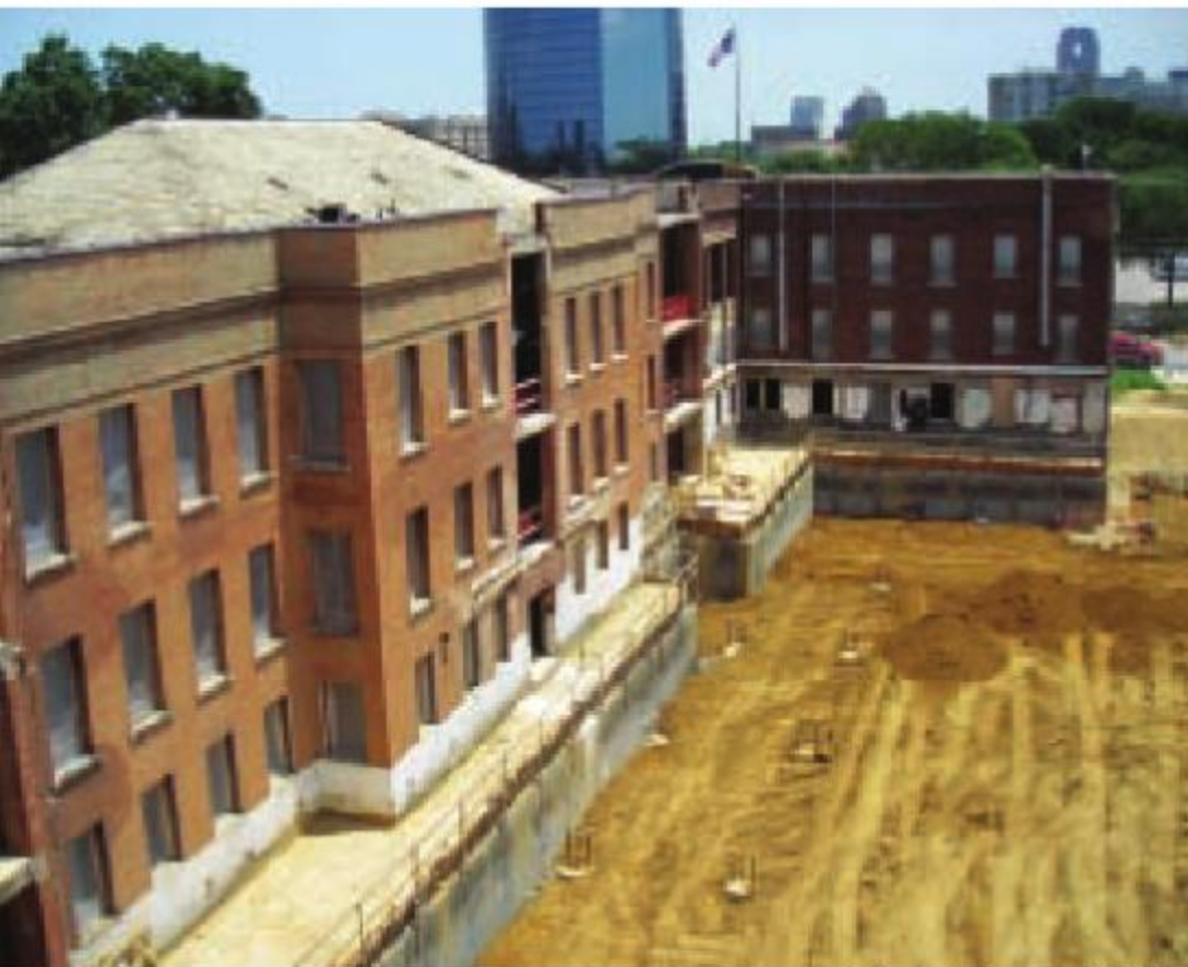
Rear View, 2007 - Good Fulton & Farrell Architects
