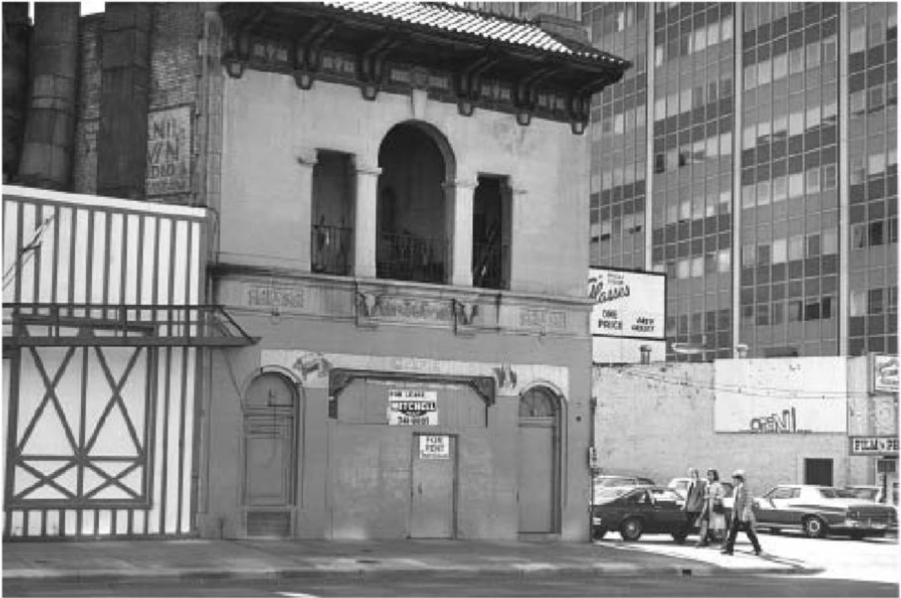
Dallas Architectural Club 1711 Live Oak Street Ralph Bryan and Dudley S. Green (façade), 1924 Demolished ca. 1980
