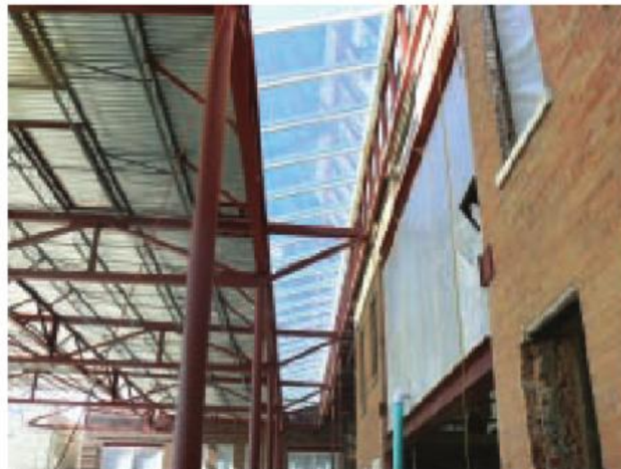
Great Room during construction, 2008 - Good Fulton & Farrell Architects
