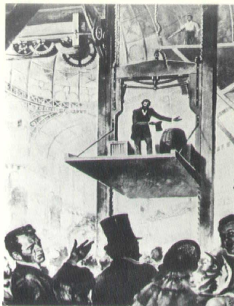
At America's First World's Fair, in the New York Crystal Palace in 1854, Elisha Otis demonstrated his safety elevator by riding on its platform as the hoisting rope was cut.
