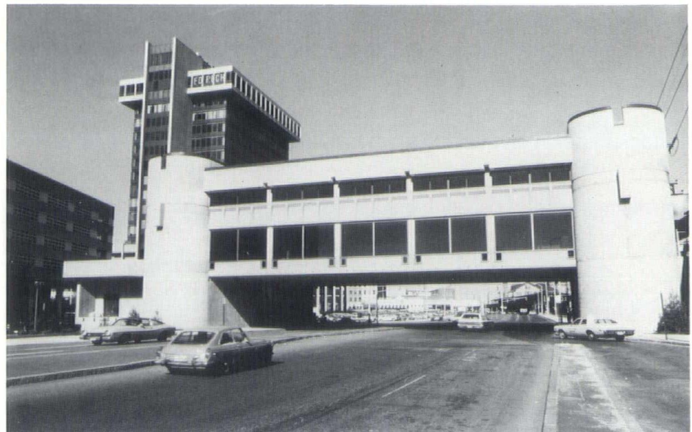
Waiting room areas and office facilities in the Bridgeport Transportation Center are located in the "bridge" spanning Water Street.
