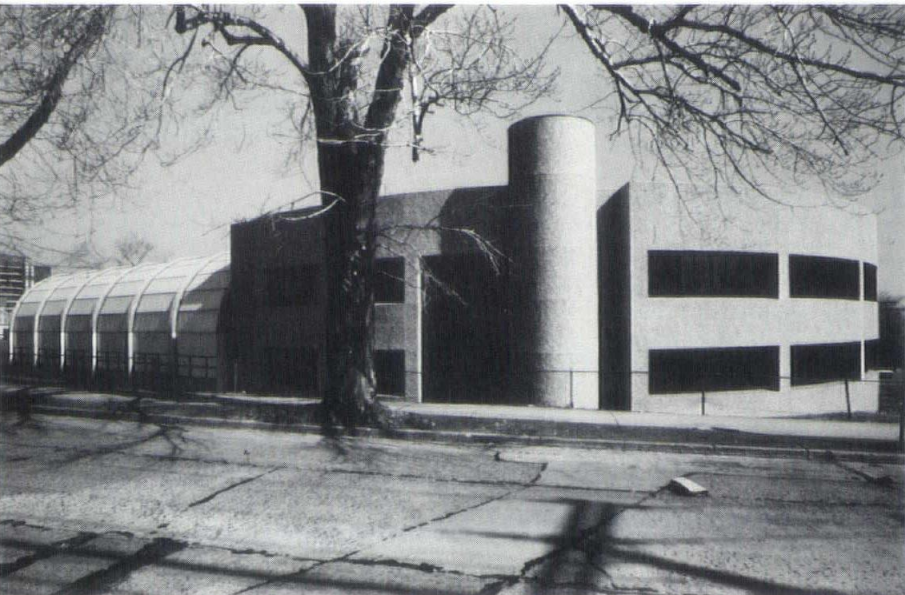
Yerwood Community Center, Stamford, Connecticut Architect: Robert L. Wilson, AIA Photographer: Martin Tornallyay
