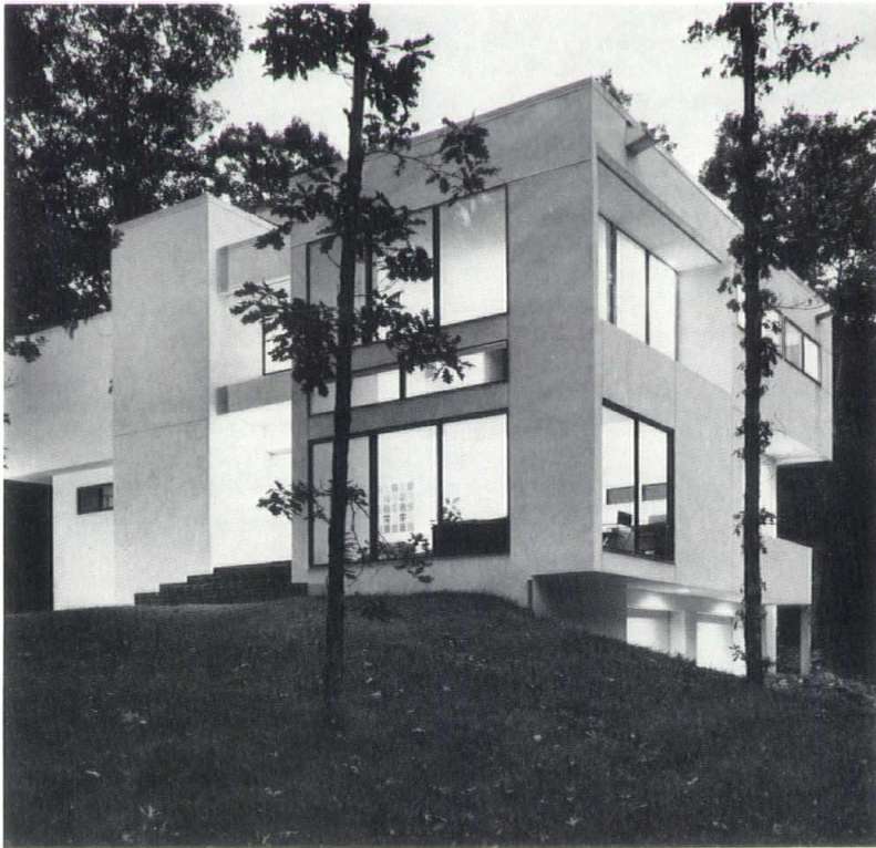
Residence, Wilton, Connecticut, Honor Award, 1974 Architect: Alan Resnick, AIA Photographer: Martin Tornallyay
