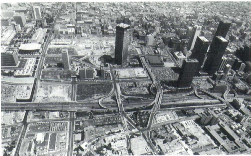
Bunker Hill renewal project in Los Angeles financed by a combination of tax increment financing and Federal financial assistance
