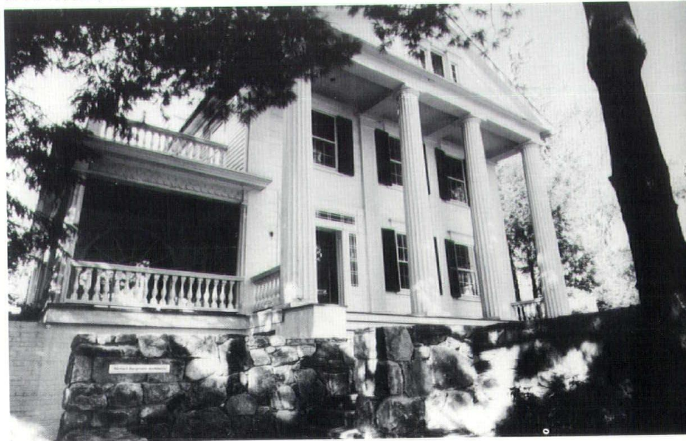
Lower level approach to front entrance on Park Street
