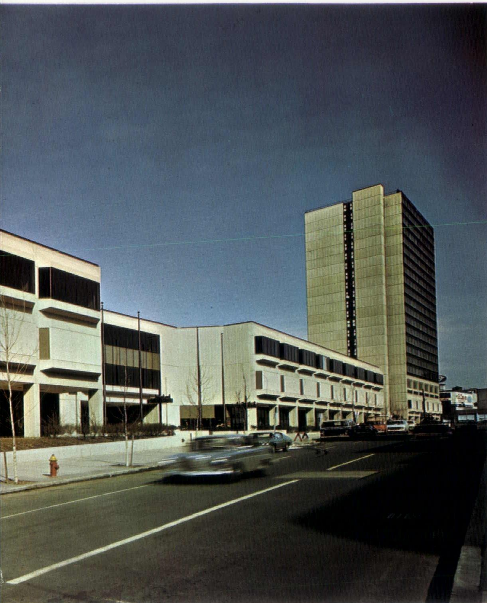
The impressive facade of the Hartford Civic Center extends from Asylum and Trumbull Streets three blocks to the new Sheraton-Hartford Hotel.
