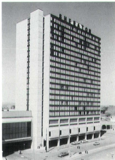
Ceco doors, frames & hardware furnished for new Sheraton Hartford Hotel.
