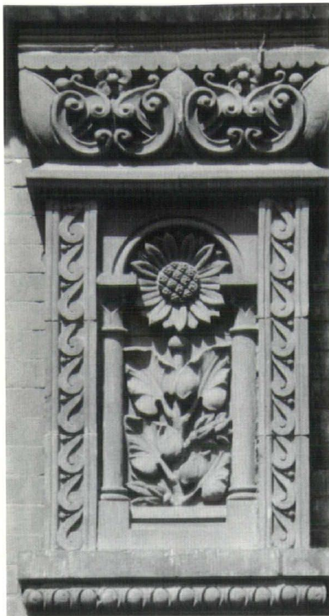
Detail of Goodwin Building, Hartford, built in 1881
