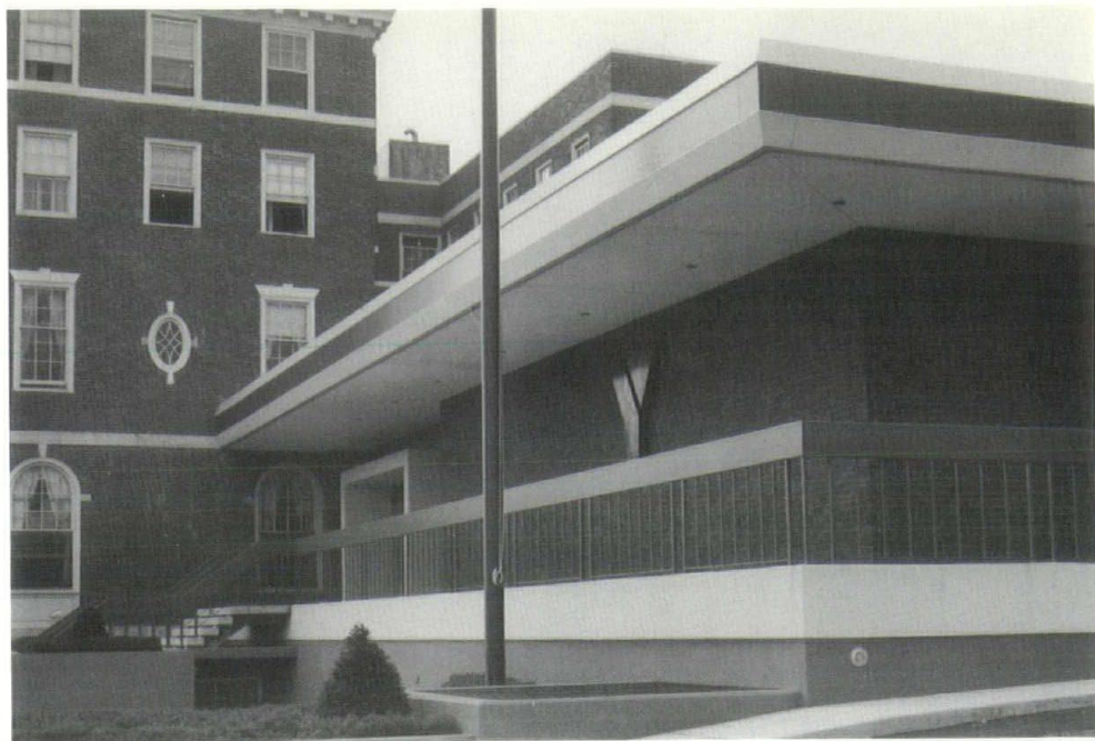
Exterior of Waterbury YMCA. Architects: Malmfeldt Associates.
