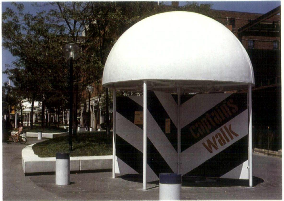
(Above) Using his navy background and design talent, Bob Steinmetz, of SMS Architects, began to give form to telephone booths, canopies and kiosks.
