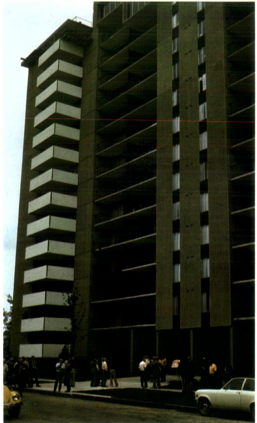
Apartment building assembled with site-cast ready mix concrete
