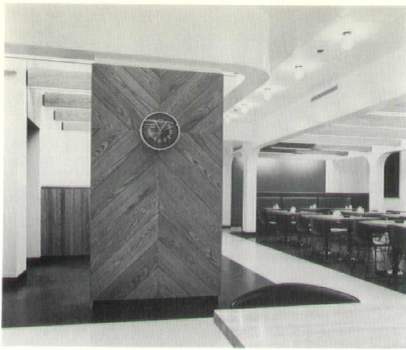
ABOVE: Free standing menu board's reverse side is paneled red oak with urethane finish worked in chevron pattern, punctuated by black and white clock. RIGHT: New dining room space developed on repetition of basic diagonal and curved lines and integrated overhead illumination.
