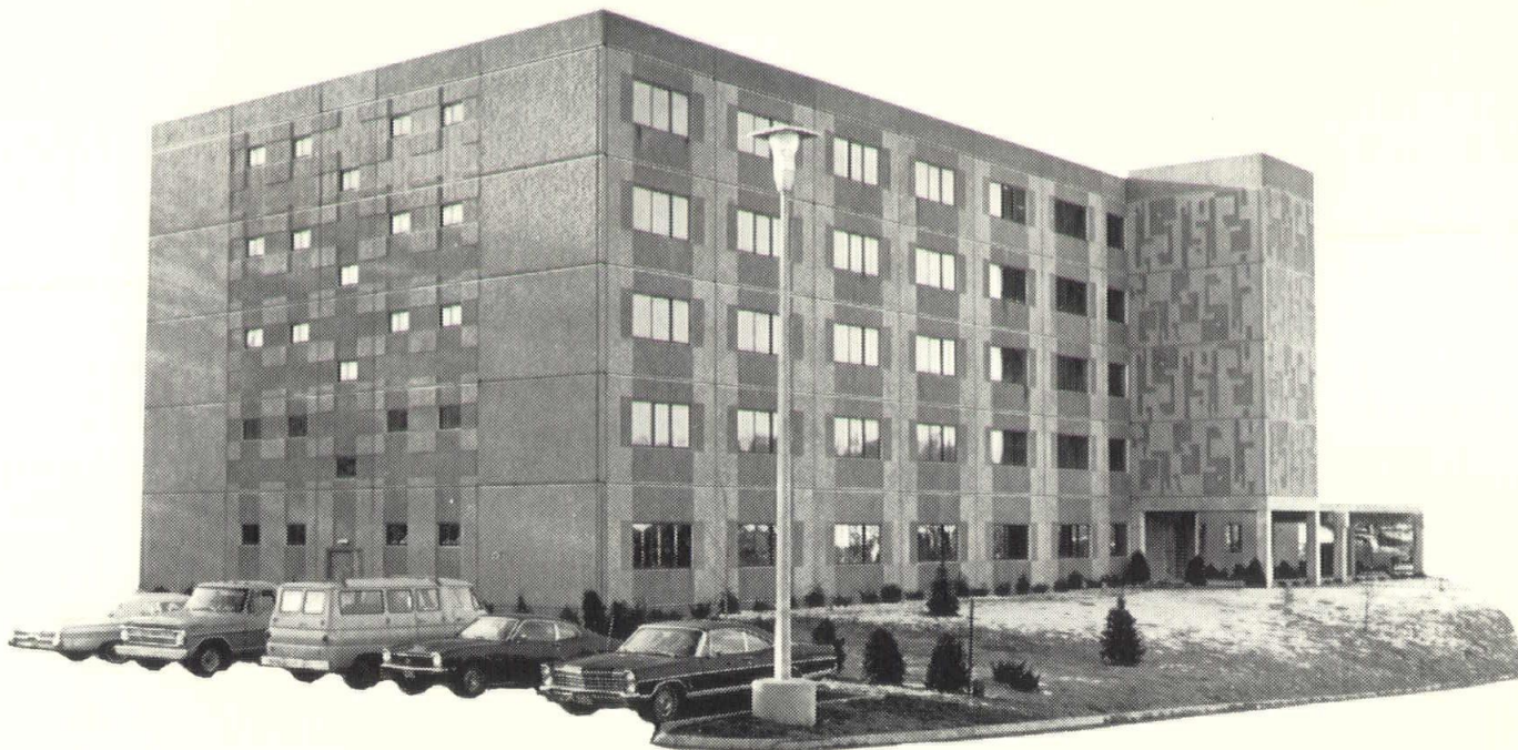
Mallview Senior Citizens Apartments, Waterbury, Conn. Developer: Michael J. Papa Associates, Waterbury, Conn. Architect: Bernard Burg, Meriden, Conn.
