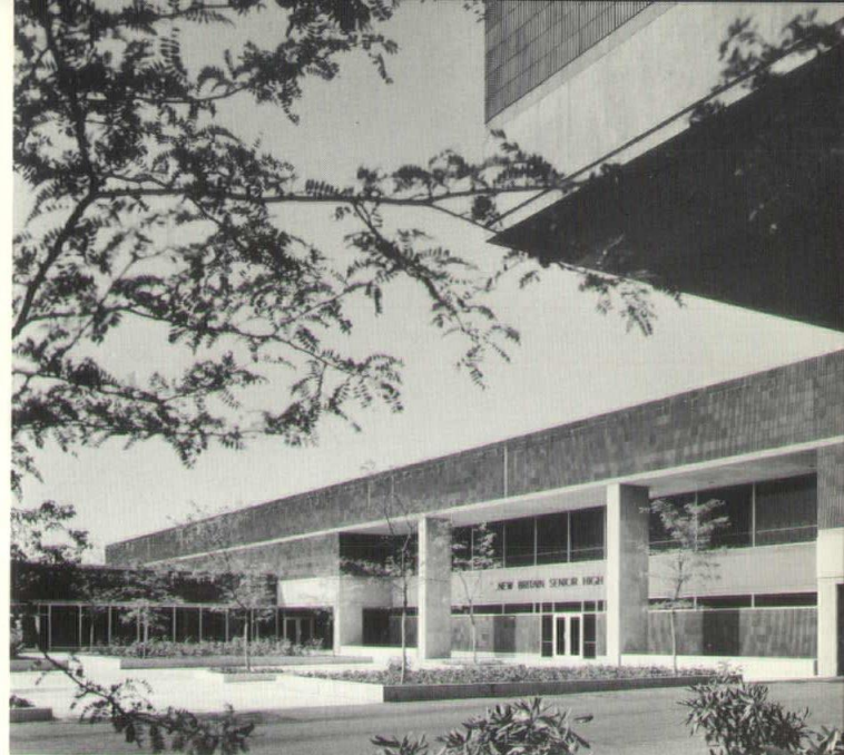
Entrance is crisp and clean.
