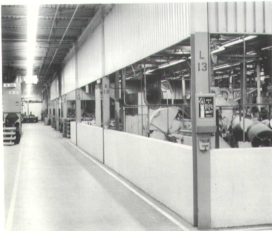
Relative temperatures are maintained in heat treating department by curtain wall.
