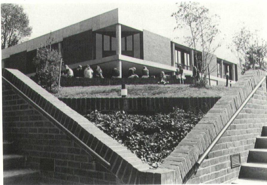
Rosemary Hall from classrooms to administration building.
