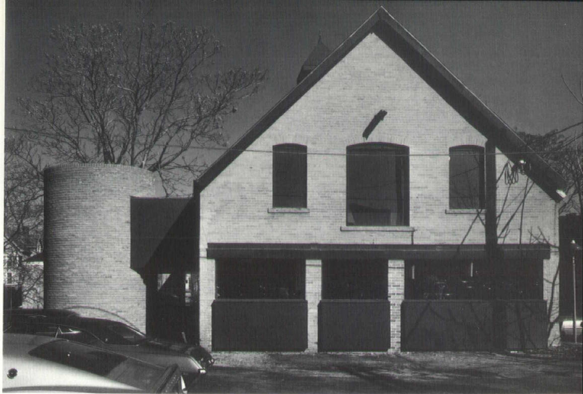
RIGHT: EDG office entrance is between silo and revitalized building in a combination which dramatizes the original crisp lines and brick facade. BELOW RIGHT: As it was.
