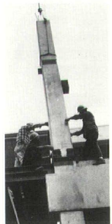
LEFT: Nearing completion, the classroom building is at the left and the resource center at the right. RIGHT: Vertical manner of construction with plant-fabricated concrete elements speeded construction.
