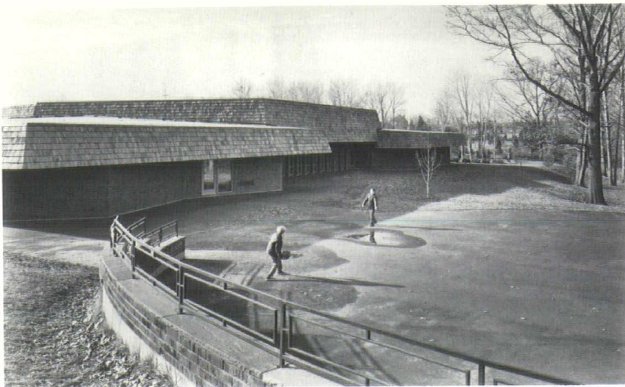
Well scaled rambling exterior is inviting to children.
