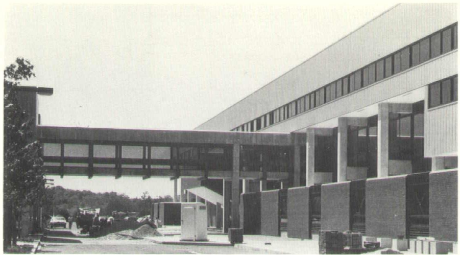
Bridge structure connects resource center to classroom building at right.
