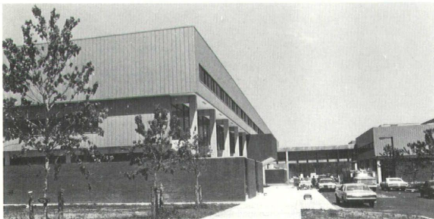
LEFT: Nearing completion, the classroom building is at the left and the resource center at the right. RIGHT: Vertical manner of construction with plant-fabricated concrete elements speeded construction.
