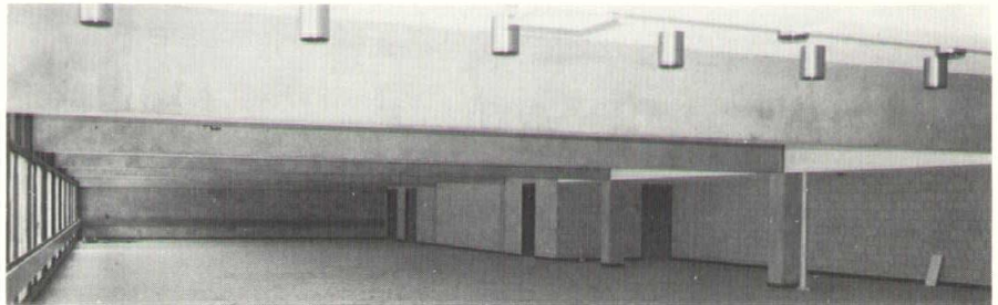
ABOVE: Long-span lines provide functional roominess in cafeteria. BELOW: Wide-span construction employed precast columns, girders, and Span-Deck flooring in classroom building.
