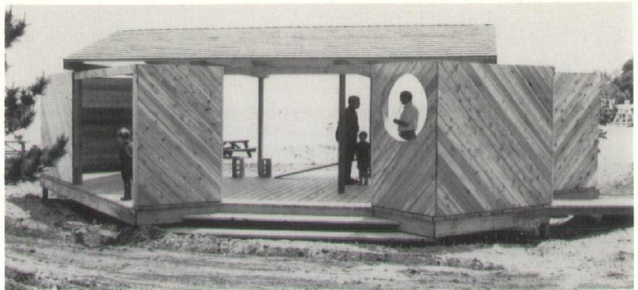
Architects, JG, inspect project.
