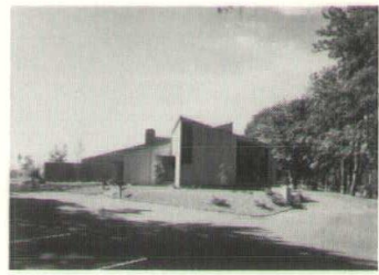
FRONT COVER: Stein Sapack & Ames architects, Waterbury designed an award winning animal hospital (page 11) which makes its owners proud and wins the approval of their clientele of pet owners. (The pets like it, too.)
