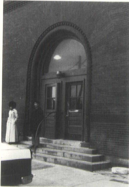
Interesting brickwork arch of main entrance of station.
