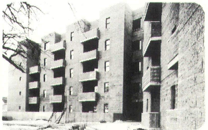
Fairhaven Senior Citizens' Housing, New Haven, Conn. — Products: Celdex® prestressed floor & roof system, profile split-ribbed facing units, precast columns and beams. — Architect: Gilbert Switzer, New Haven, Conn. — General Contractors: Giordano Construction Co.
