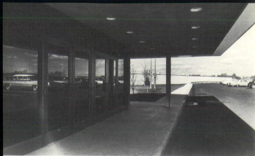
Protection from weather is main entrance feature.
