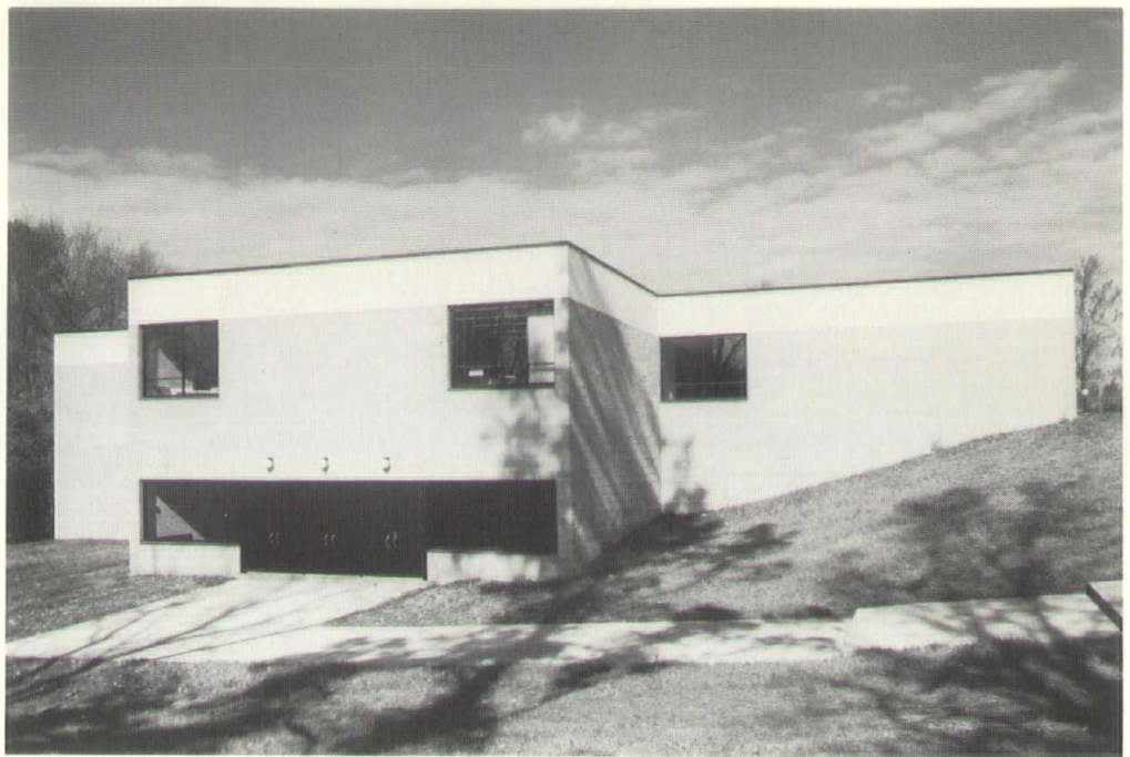
Lower level entrance.
