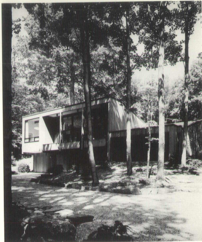
House fits naturally in sloping site.
