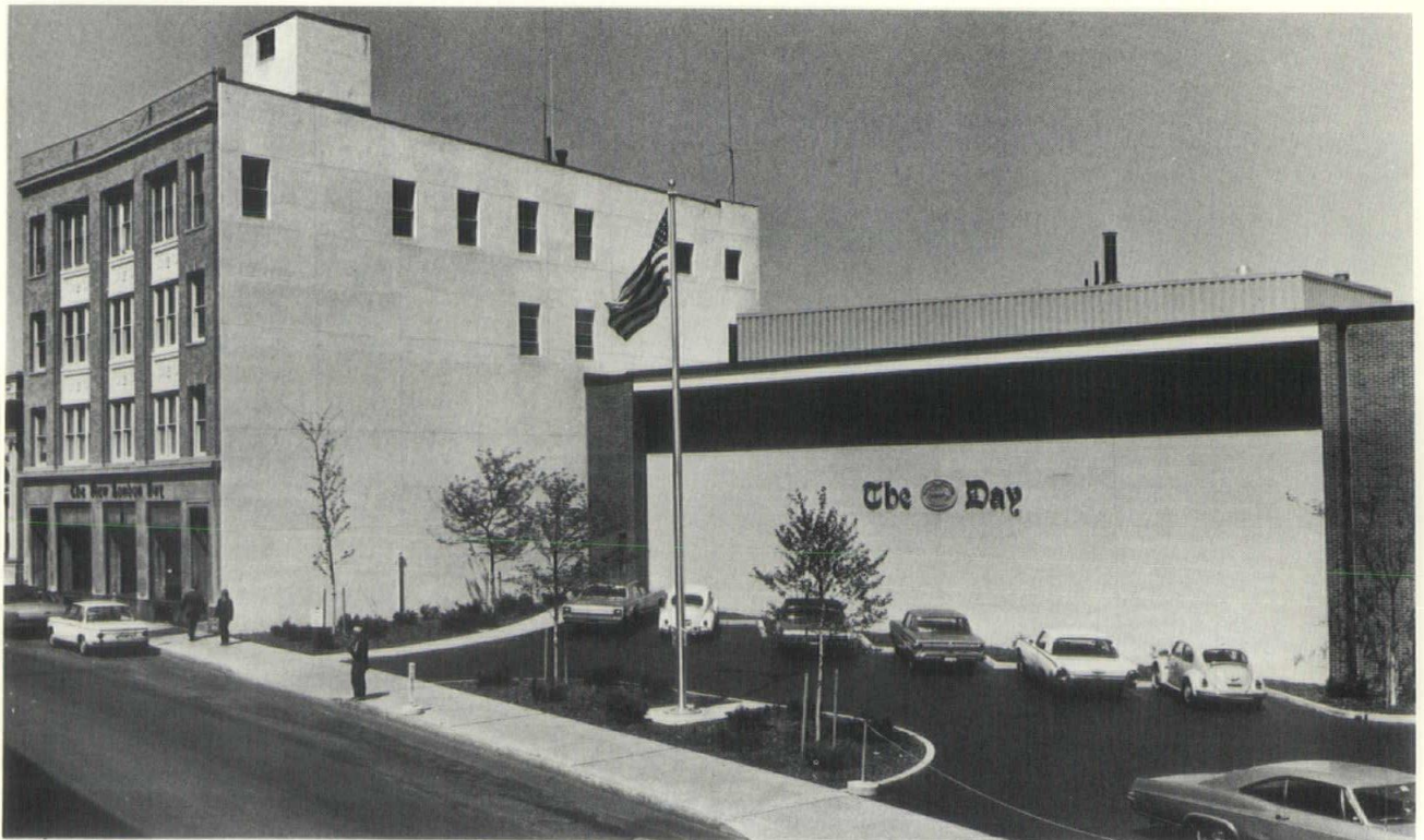
New addition and existing building.
