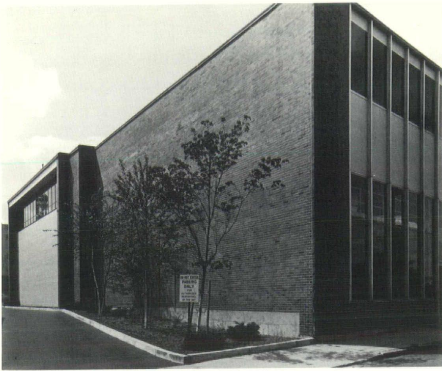
The new building (at the rear) joins naturally with 1961 addition in foreground.
