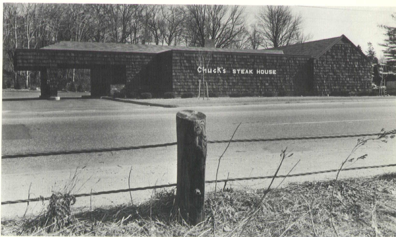
The new Chuck's Steak House. Wood parapets conceal copper gutters; cantilevered overhang of auto canopy permits two cars to unload in foul weather.
