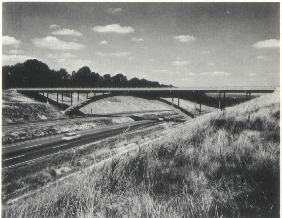
This Connecticut highway bridge spanning Interstate 84 in Middlebury won an American Institute of Steel Construction Design Award.
