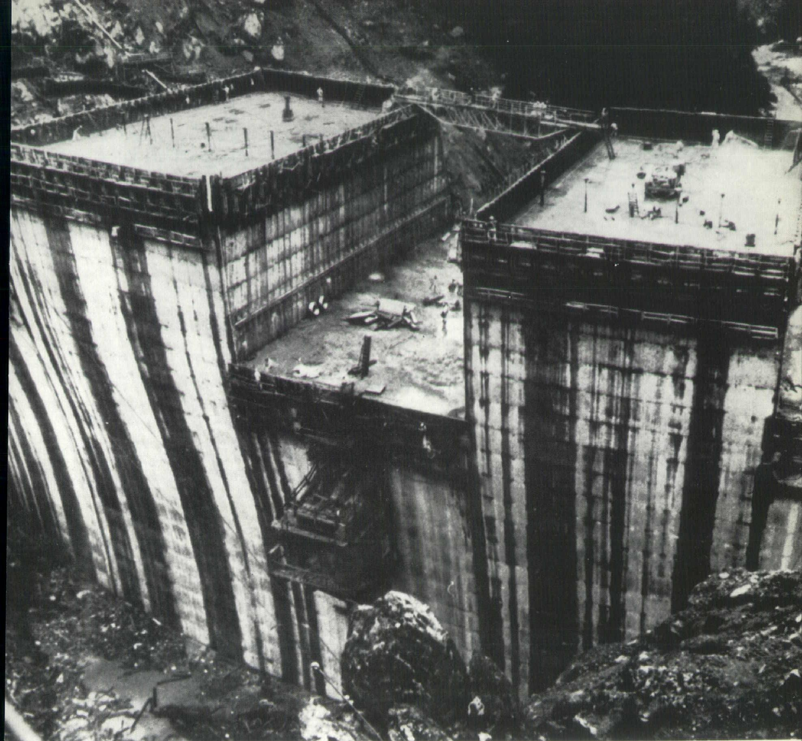
Yuba River Development Project, Dobbins, California. Contractor: Perini-Yuba Associates.
