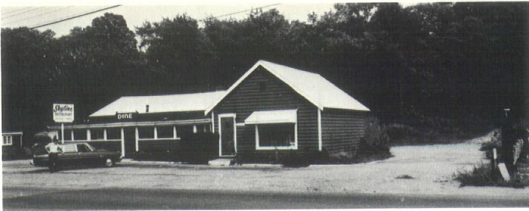
Building before renovation, ordinary and uninviting.
