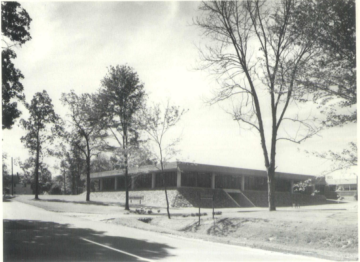
The building appears to have "grown" on the site.
