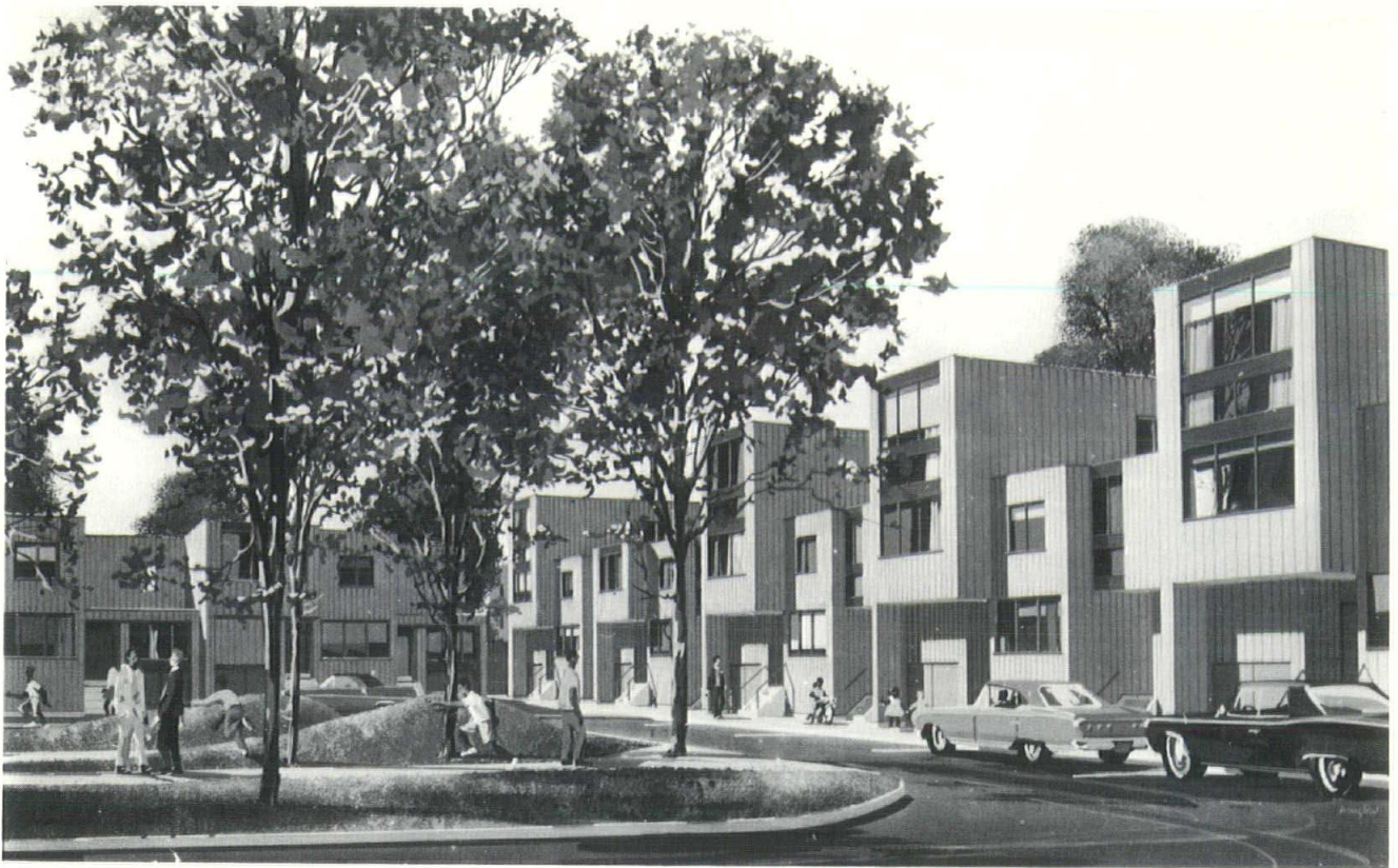
Low and moderate income housing (22 units—1969), Dwight Project, sponsored by Congregation Beth Israel; Louis Sauer, Architect.
