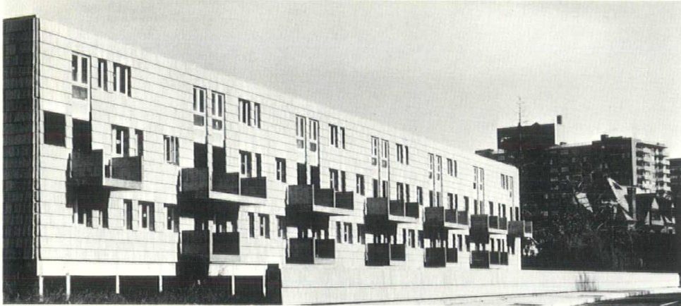
Columbus Mall, moderate income housing cooperative (72 units—1964), sponsored by Hershman Foundation; Earl Carlin, Peter Millard, Architects.
