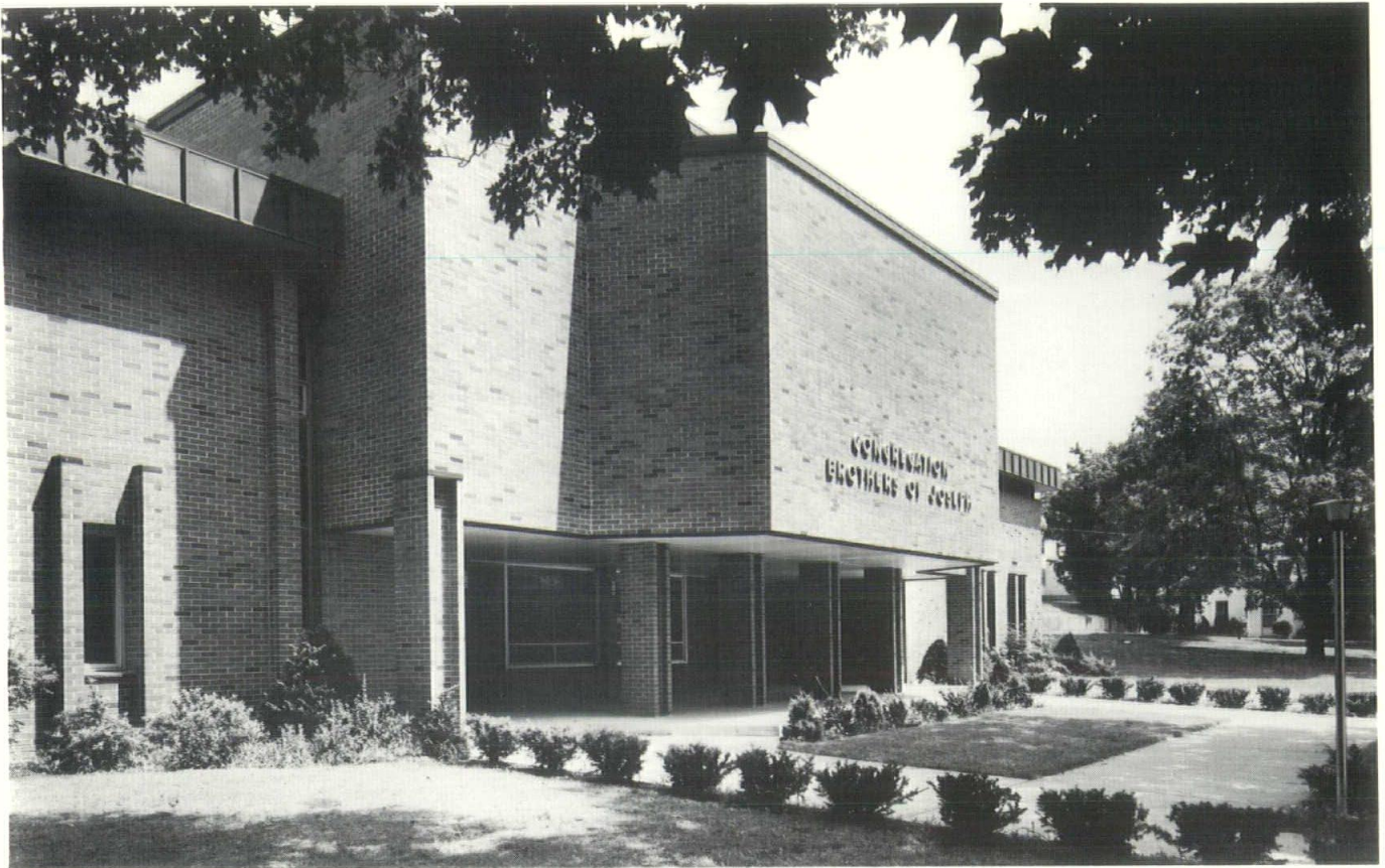
Lower level entrance.
