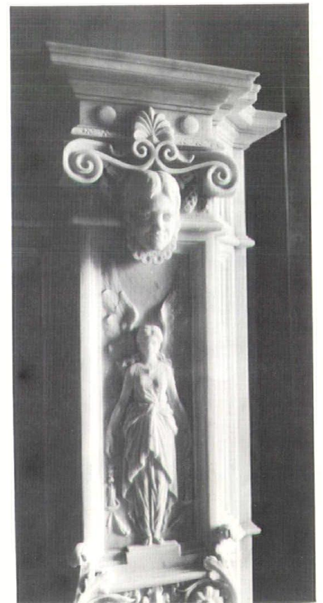
Detail of drawing room mantel, carved by hand in solid marble, is typical of the craftsmanship in the mansion.
