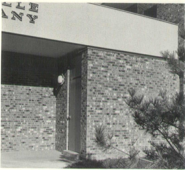
Rear entrance detail.
