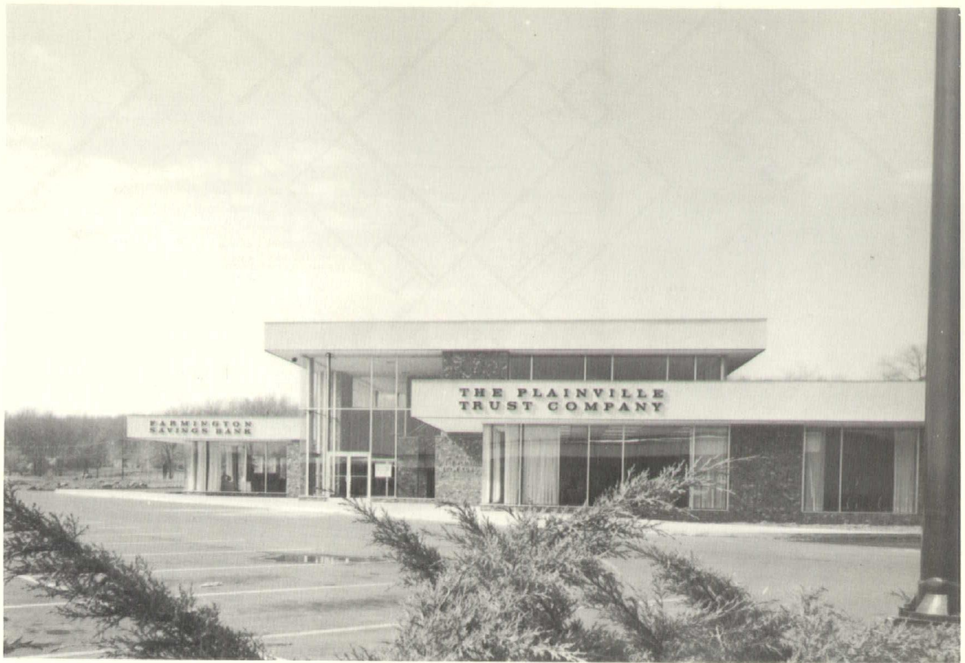
Bank building dominates entrances to shopping center.
