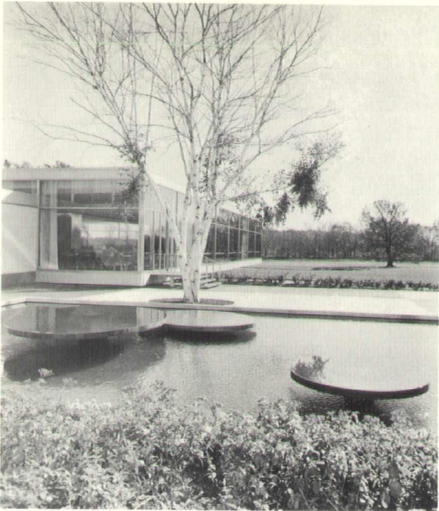
Three sculptured cast concrete, bronze rimmed lily pads, by Noguchi, lend an added dimension to the reflecting pool off the South Terrace of Connecticut General's home office building. In the background is the Company's cafeteria.
