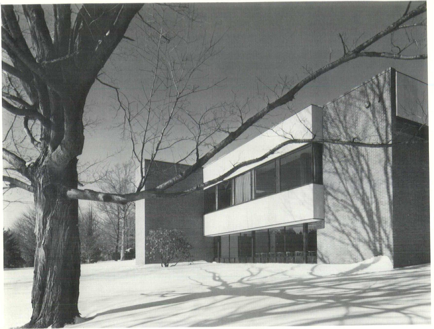
Glass and brick combine in strong, simple facade.
