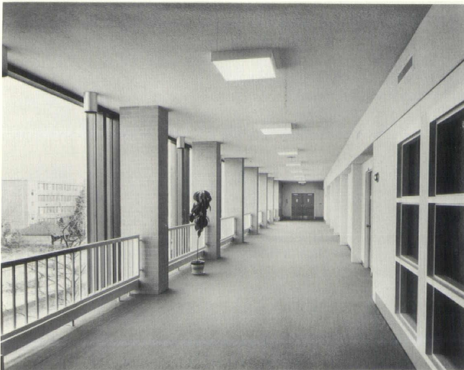
Main circulation areas are at front of building.
