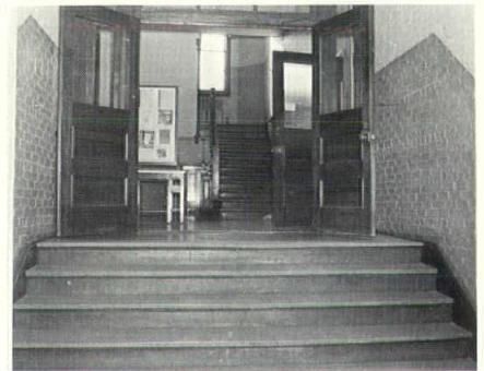
Before and after alterations, showing new main floor reception area in Gulley Hall.
