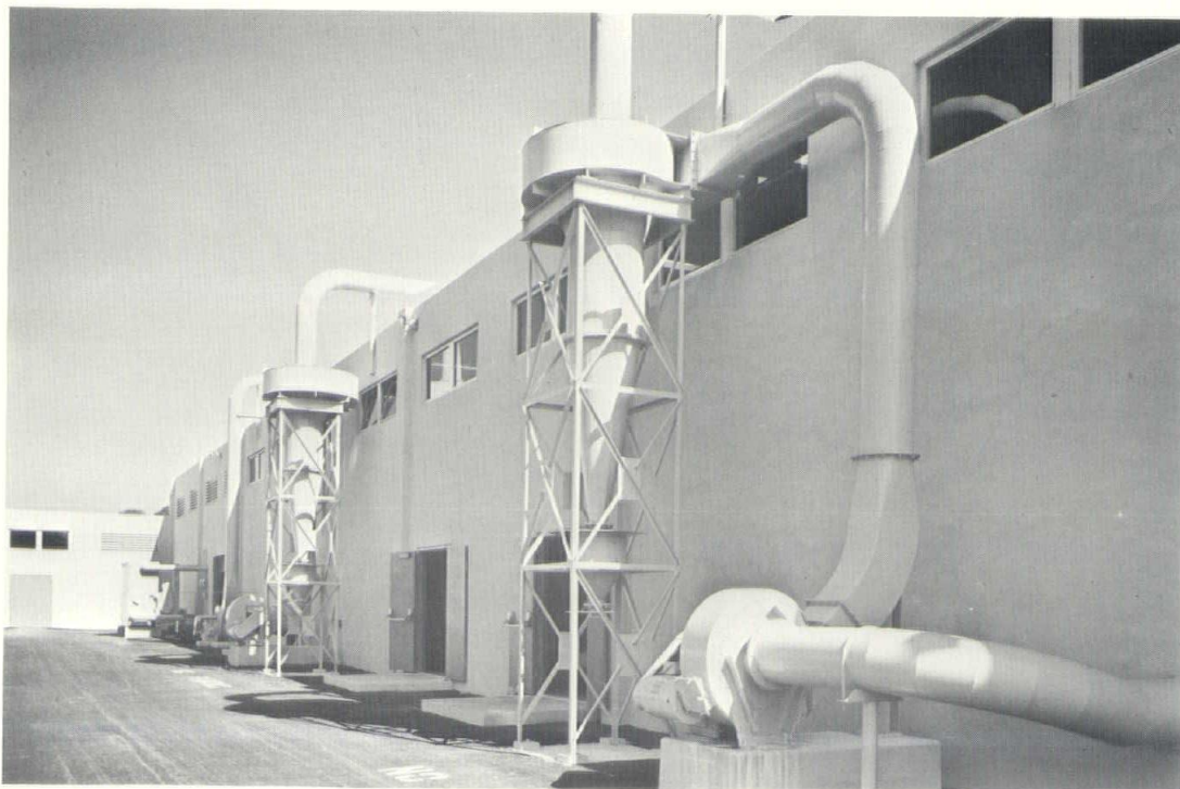
Cleaning equipment placed outside facilitates servicing and frees interior space.
