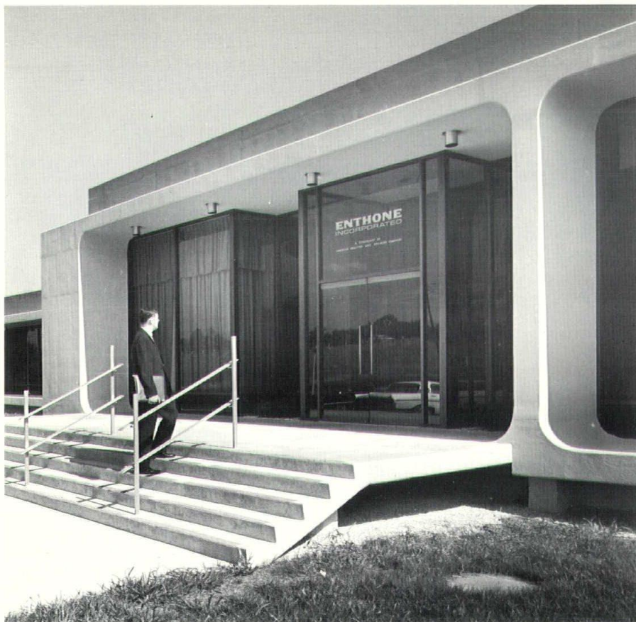
Imposing main entrance is focal point of facade.
