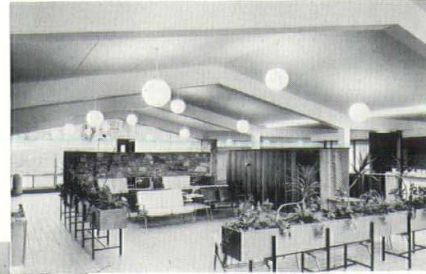
SPAN-DECK Precast Prestressed Concrete Roof Deck Used Completely Exposed as Finished Noise-Reductive Ceiling
