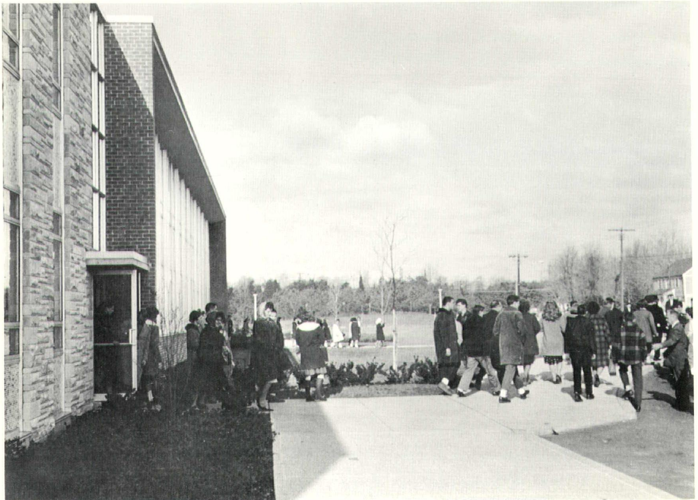
Opening day and the school is ready.
