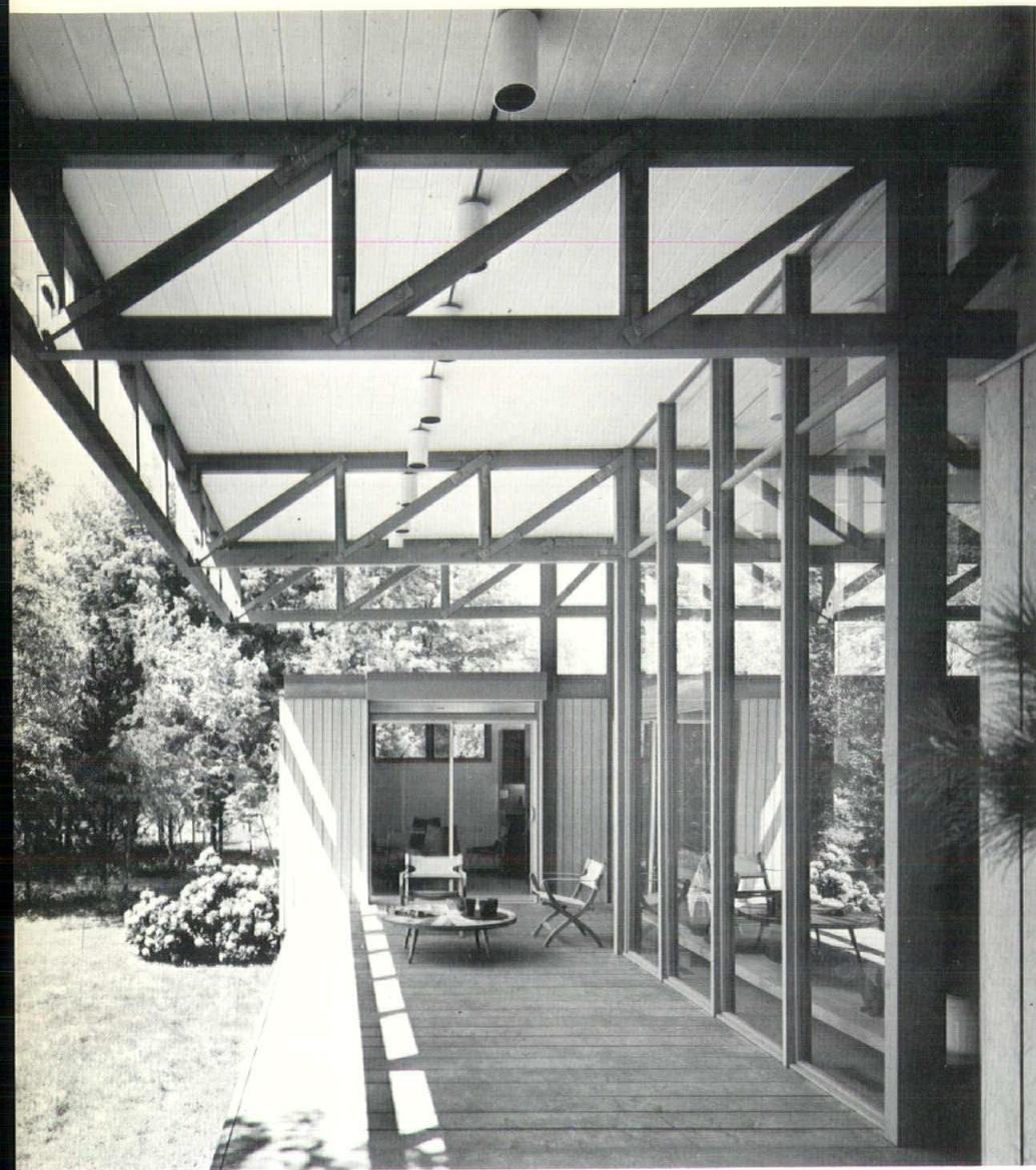
Deck, an extension of interior floor, is reached by sliding doors at sides of fireplace and from breakfast area.
