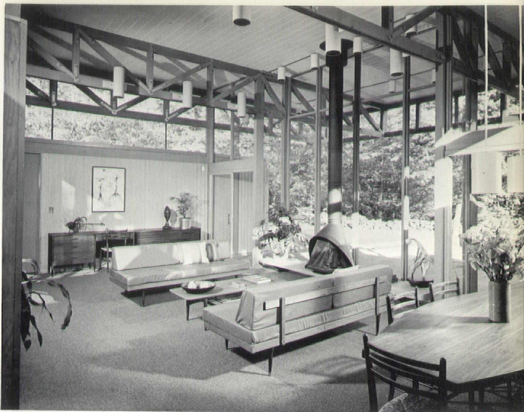
Lighting is designed to provide variable effect in all areas.
