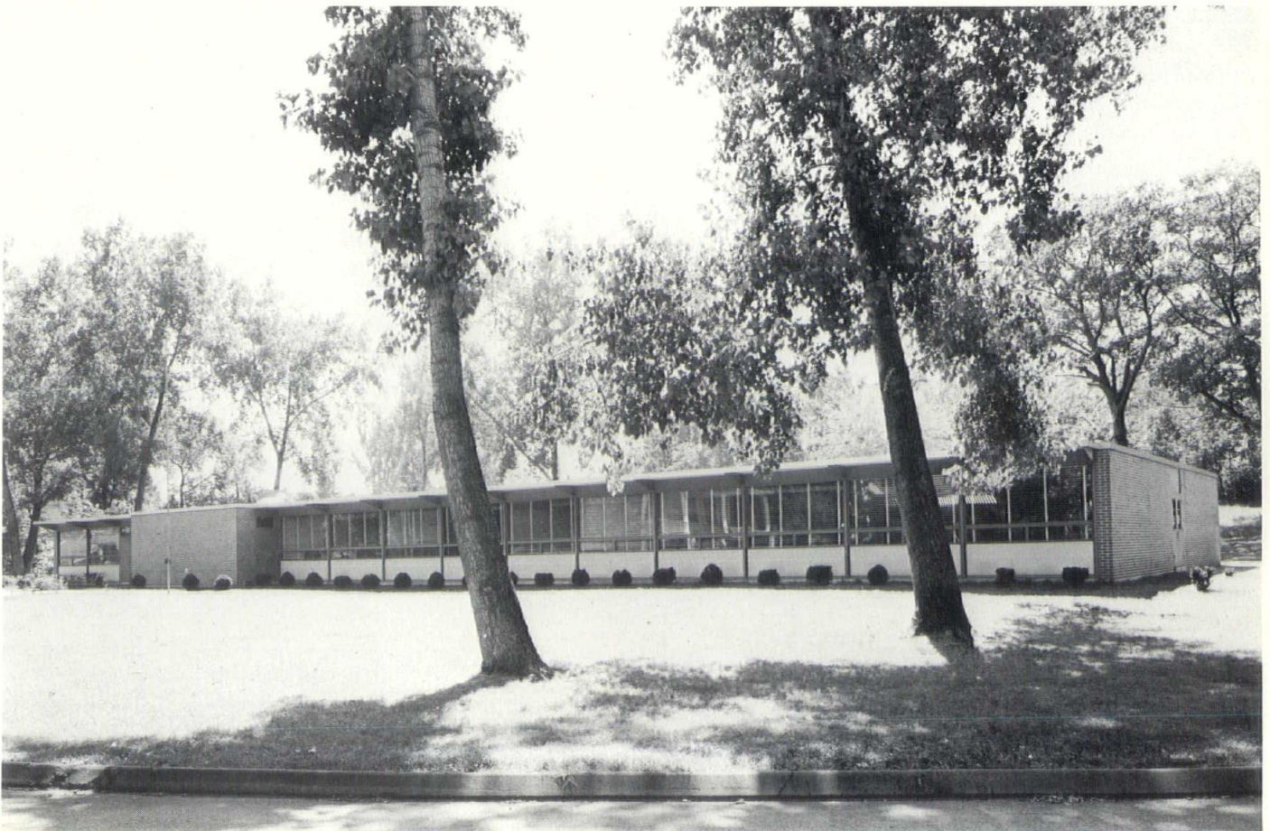
School building faces residential street.
