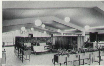
SPAN-DECK Precast Prestressed Concrete Roof Deck Used Completely Exposed as Finished Noise-Reductive Ceiling
