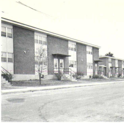
While buildings adjoin each other closely on both sides of streets,
