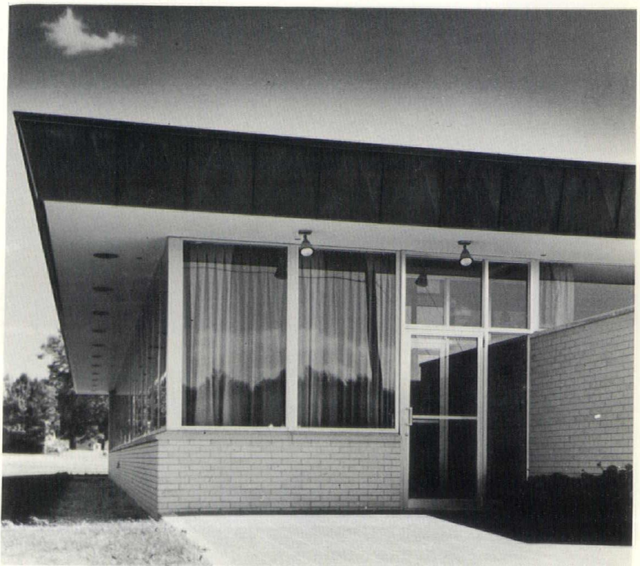
Entrance to office showing overhang and placement of exterior lighting fixtures.
