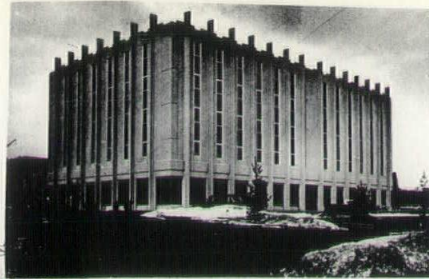
DOCTOR'S BUILDING Architect-Engineer Westcott & Mapes, Inc.
