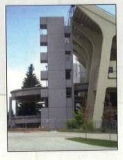
Four vertical precast Super Columns, each 100 feet in height & weighing 240,000 lbs provided the structural support for the new luxury suites & indoor club level seating
