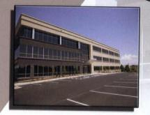
100,000 SF of total precast core and shell Total production 681 pieces Total erection time 48 days
