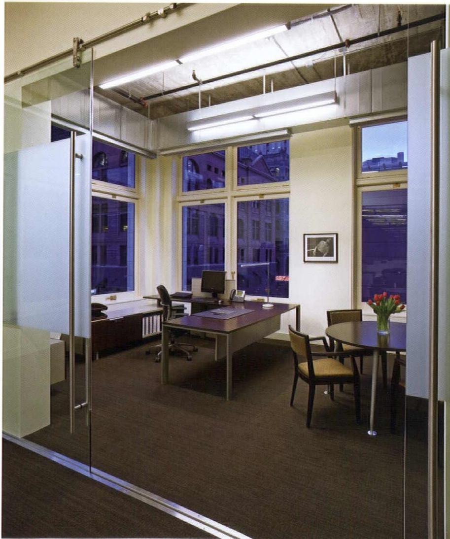
Below: Windows on the front façade proved to be a test of the project’s mettle; the eventual solution maintained their profiles and unique pivot within a new energy-efficient window system.
