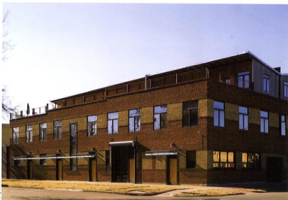
Above: Conversion of a furniture warehouse into residential lofts. The original building was divided into 10 3-story lofts. The existing building perimeter was selectively perforated to create doors and windows appropriate for residences.
