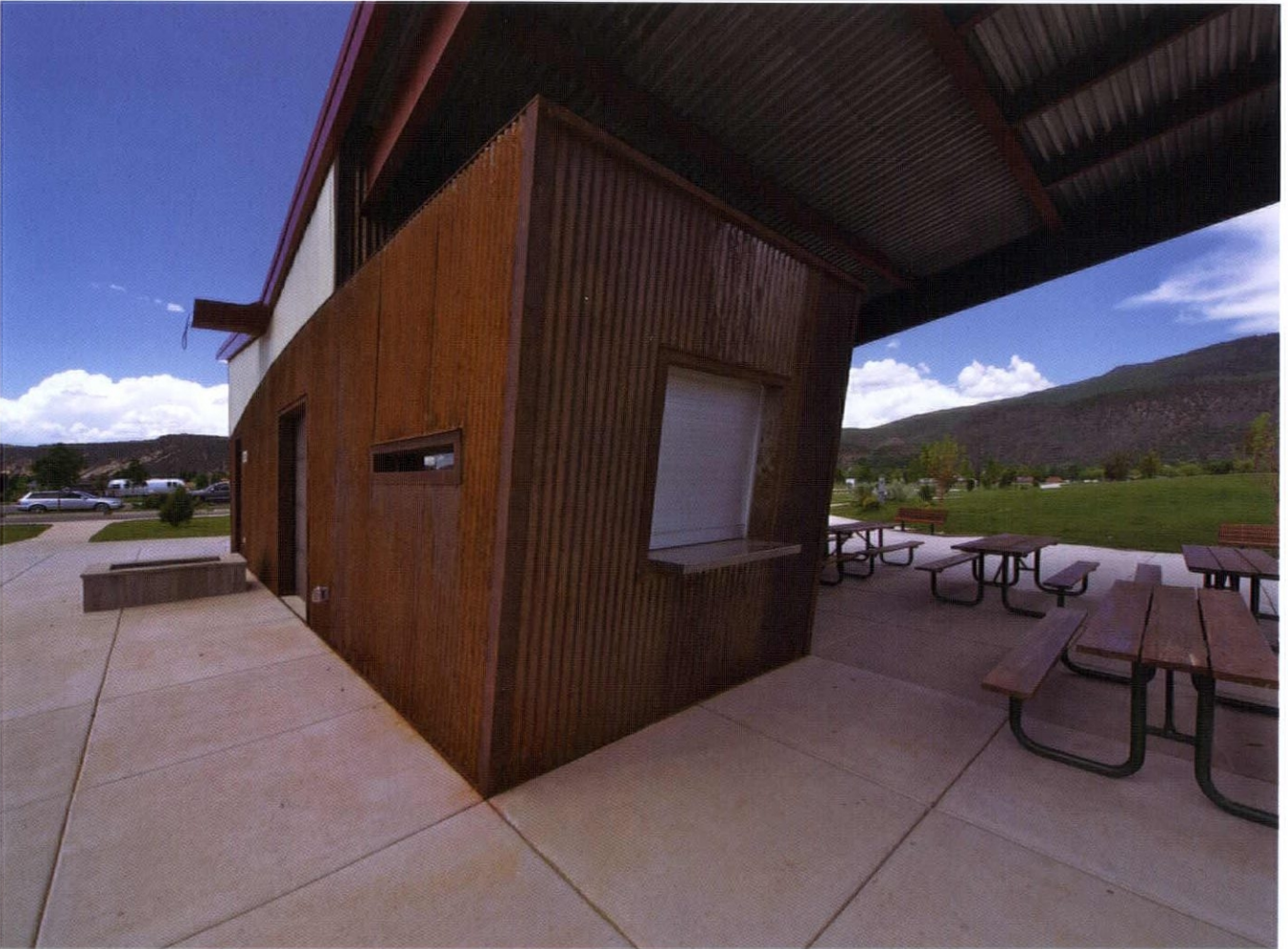
An oblique view of the concession area that has shipping container massing and is neatly sheathed in rusted non-galvanized corrugated steel. The building components are placed at opposing angles resulting in a rich, textural composition of layers and shadow.
