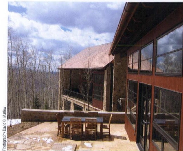
Above and left: Dominick designed the Mountain Star residence in Avon, Colo., as a series of three stone "cottages," all detailed in a similar manner. The sections are linked by steel and glass greenhouses. The top cottage at Mountain Star was aligned with the site to reduce the side hill excavation; the remaining two were aligned across the contours to provide 180 degree mountain views.
