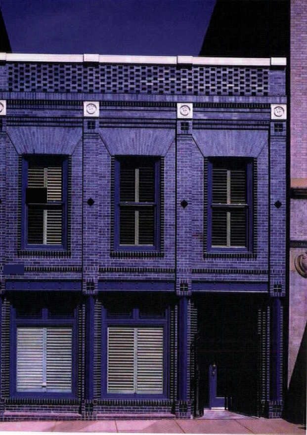
Above and below: Dominick incorporated brick, painted steel and punched glazed openings into the exterior design of Denver's Cactus Club, weaving new technology with traditional materials. The great hall in the building is lit by a series of clerestories.
