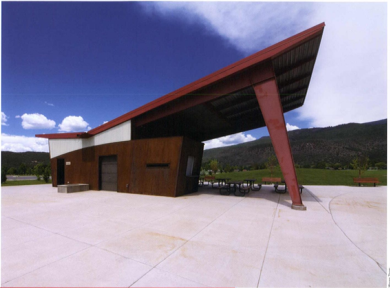
Above: The exposed tapered steel plate girders and dramatic sweeping roof of the concession facility at Crown Mountain Park recall the drive-in genre of the '50s. The project received a 2008 AIA Colorado West Citation Award.
