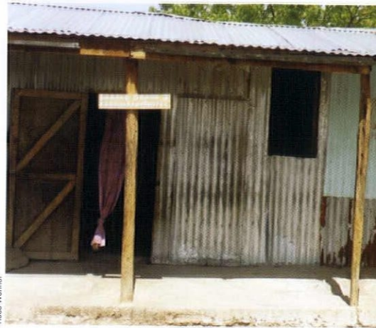
Photograph of an existing building at The Shompole School for Girls.
