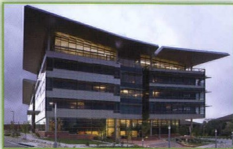
Signature Centre at Denver West, LEED Platinum Building
