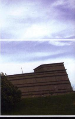
REMAX INTERNATIONA HEADQUARTERS The 850-car Parking Structure Podium is composed of 225,000 SF structural precast framing with architectural precast load bearing wall panels. The precast architectural wall panels consisted of a three-different-aggregate blend to simulate and complement the granite used on the Office Tower.
