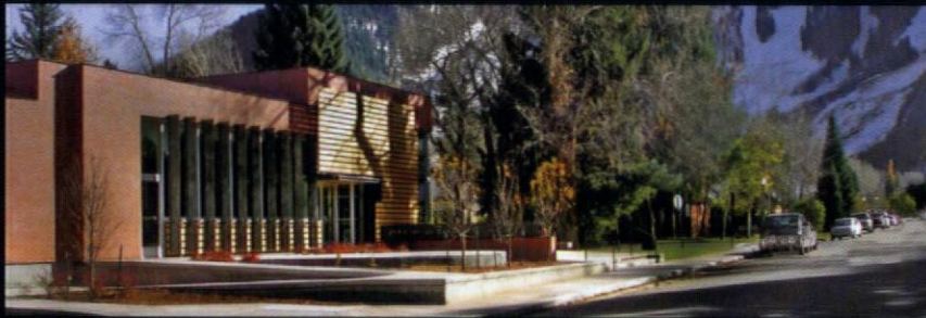
Red Brick Center for the Arts Aspen, CO
