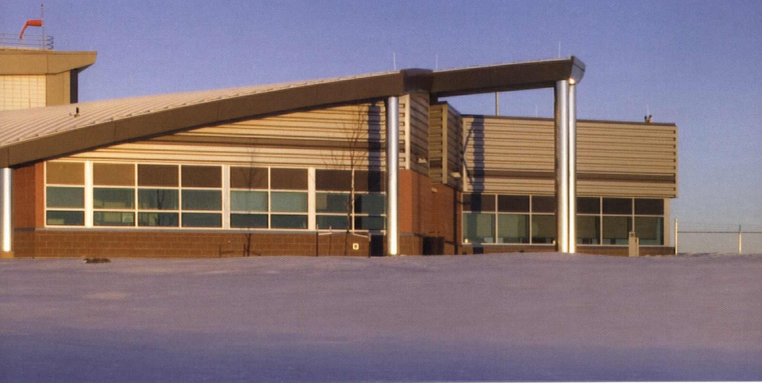
The soaring shape of the exterior references a helicopter blade.
